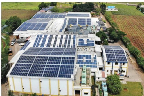
SOLAR PANELS OCCUPYING ROOF SPACE. ARIEL VIEW OF DOMAIN DINDORI, OUR LARGEST FACILITY
